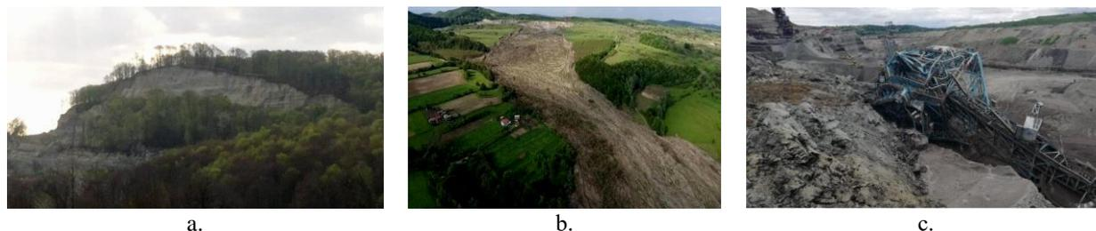
Fig. 1. Slope slides; a. Ruget open-pit; b. Berbești West external dump; c. Olteț – Alunu open-pit
